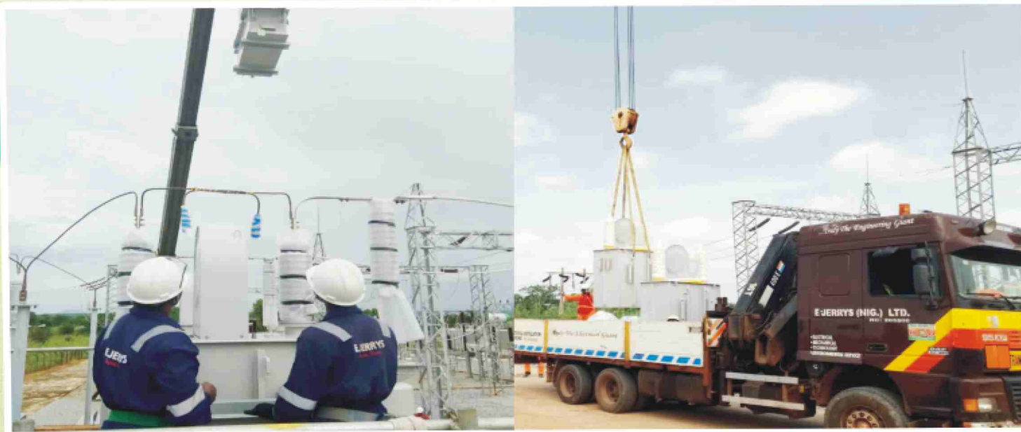
Assembly of 26MVAR Reactor
