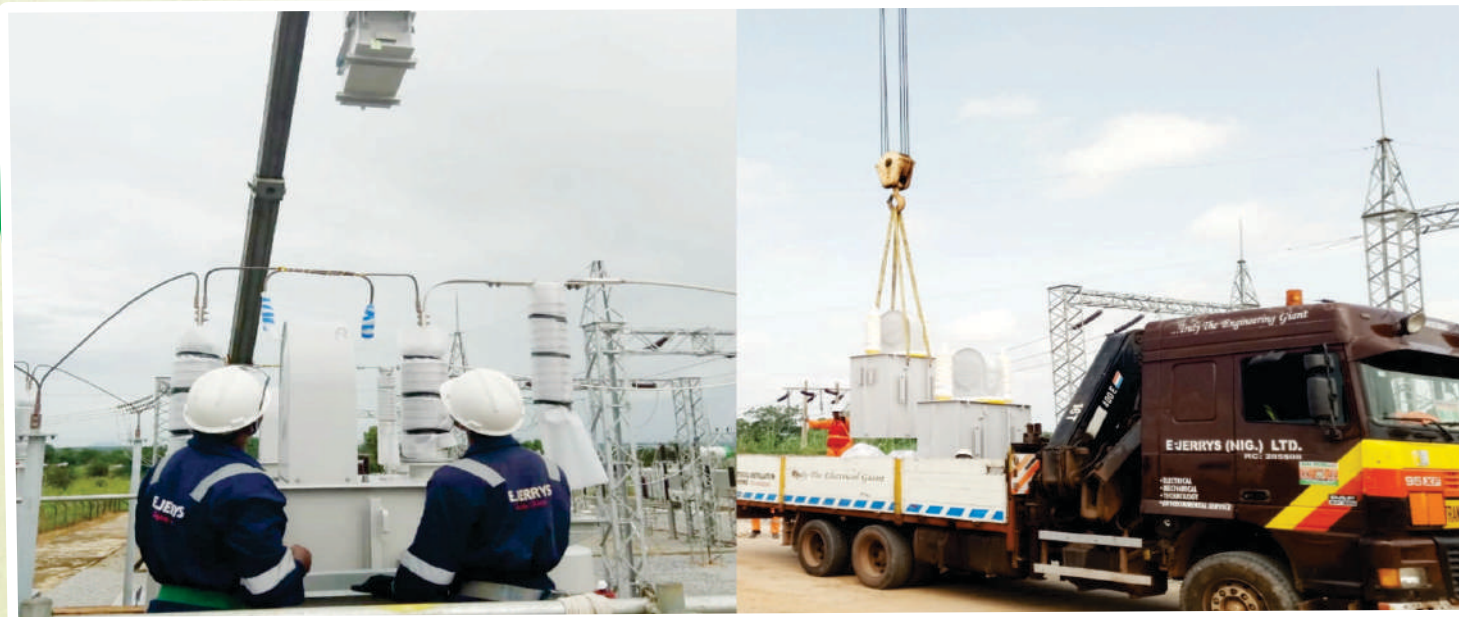
Assembly of 26MVAR Reactor
