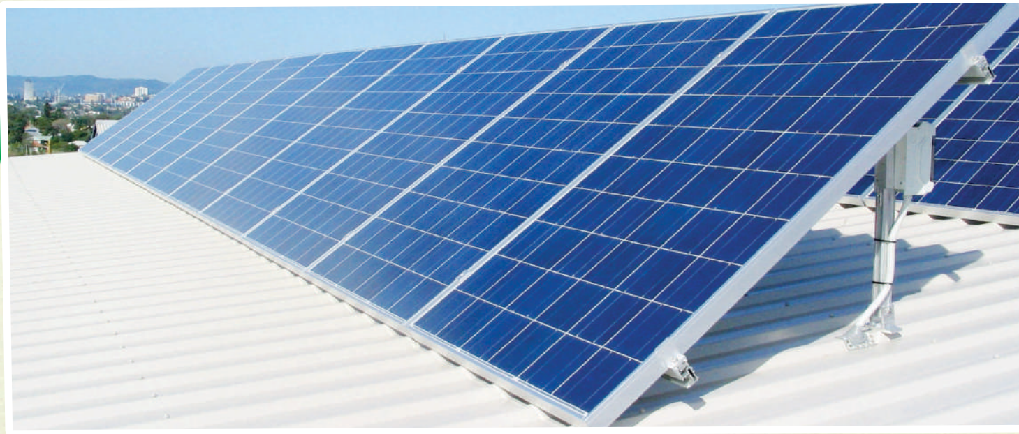
Solar Panel Installed
